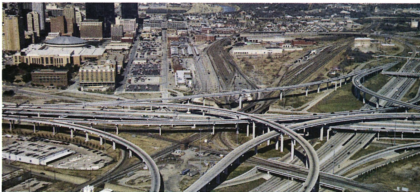
The Mixmaster, Fort Worth. This is where I-30 and I-35W meet, but if you look closely you can see the historic junction below the highway, where several major railway lines have met since 1881. From Historic Texas from the Air , by David Buisseret, Richard Francaviglia and Gerald Saxton. Aerial photographs by Jack W. Graves, Jr., published by University of Texas Press.
